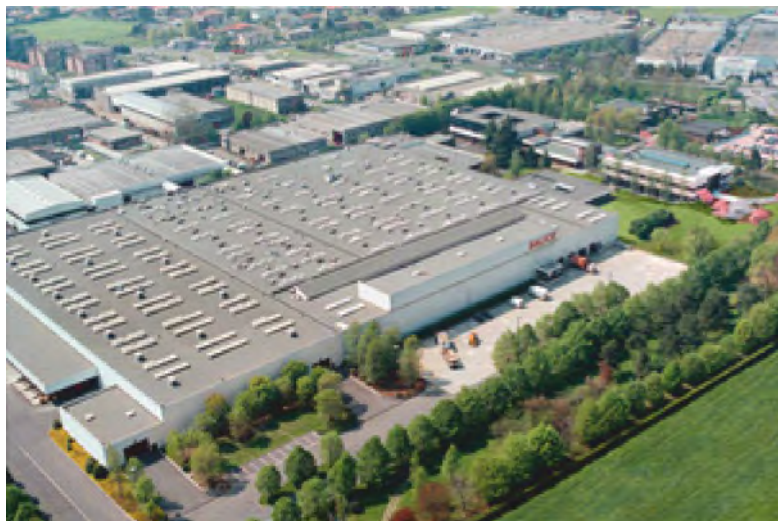
View of the Salice Factory in Italy.
